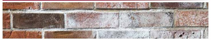
Efflorescence is a white, crystalline substance that can appear on many building materials (including stone veneer, bricks, cement walls, grout and fiber cement). Although uncommon, efflorescence may occur within TruExterior® Siding & Trim products.
